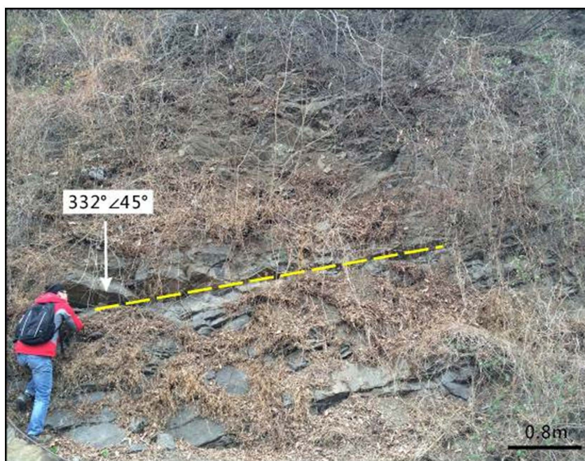
Figure 1. The shale in front of the landslide
